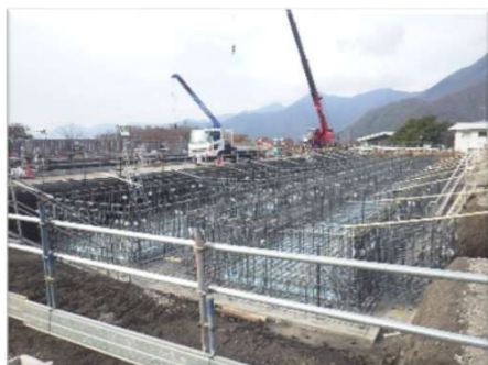
宿泊棟基礎配筋
